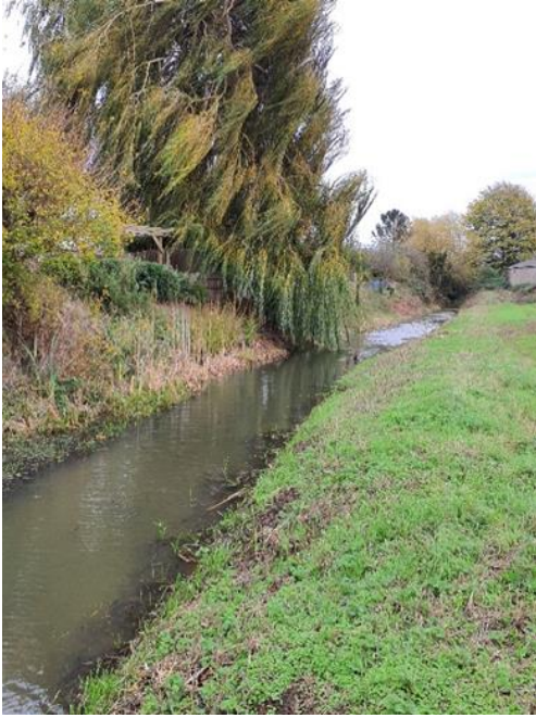
Photo 4-39: Old Trent Dyke Cullen Close
