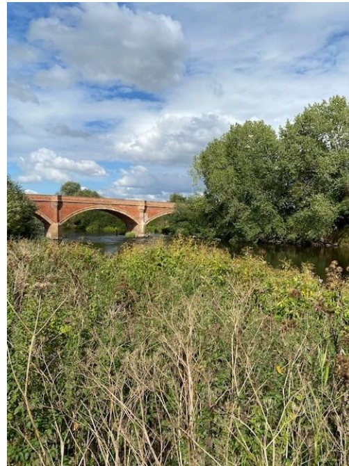
Photo 4-2: KC3 module 5 facing downstream
