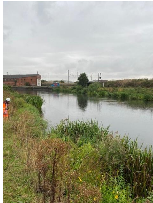
Photo 4-22: MC5 module 2 facing downstream
