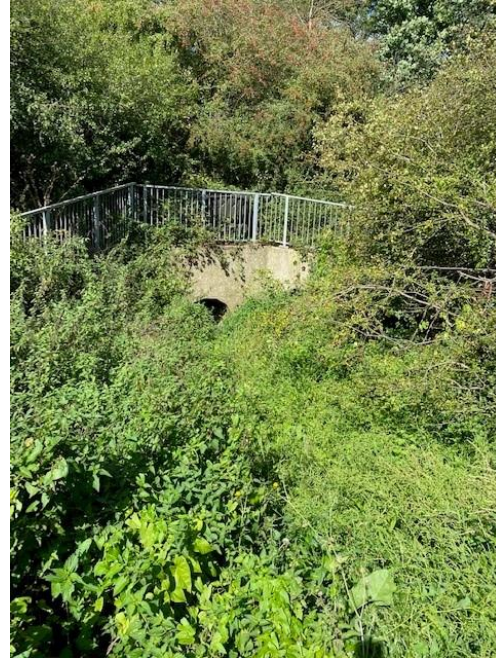
Photo 4-44: Old Trent Dyke River Trent to A46
