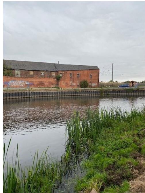
Photo 4-18: MC5 module 3 facing downstream
