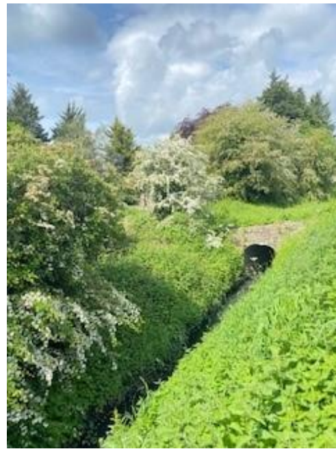
Photo 4-32: SD3 module 4 facing downstream
