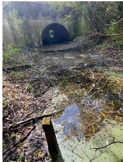
Photo 4-42: Old Trent Dyke A46 culvert
