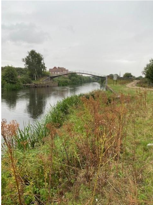
Photo 4-19: MC5 module 2 facing upstream
